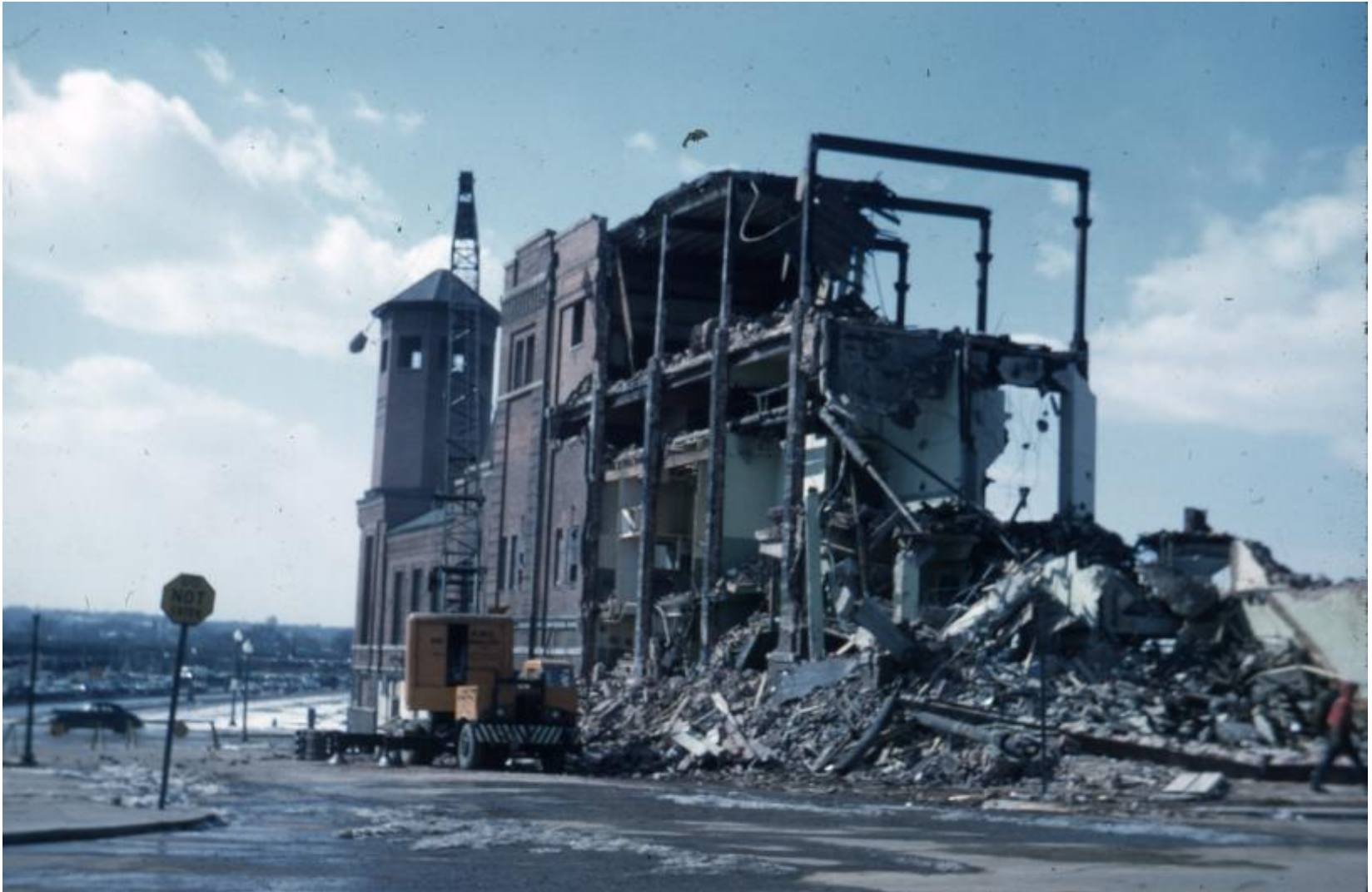
The Waterfront Carillon and the storage warehouse came down one wintry day. The big crane, swinging the giant “pear”, banging away
