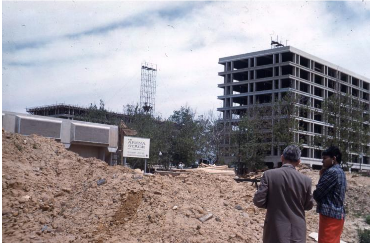
The Arena Stage under construction – CULTURE! Good luck to it! And more apartments.
